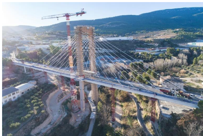
Image Property of FCC Construction
