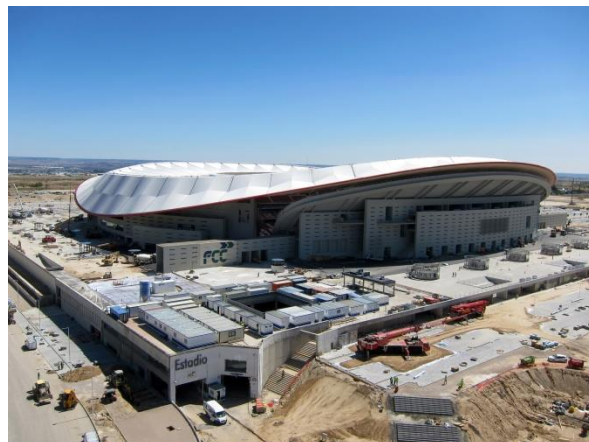
Image Property of FCC Construction
