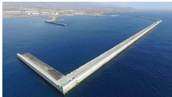
Image Property of FCC Construction
