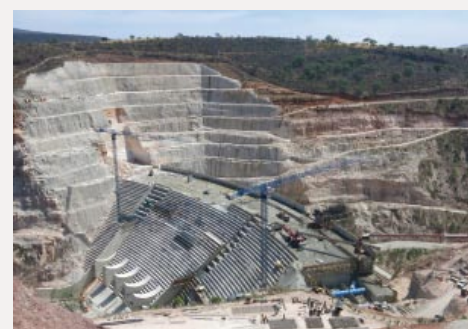
Zapotillo Dam, Mexico
