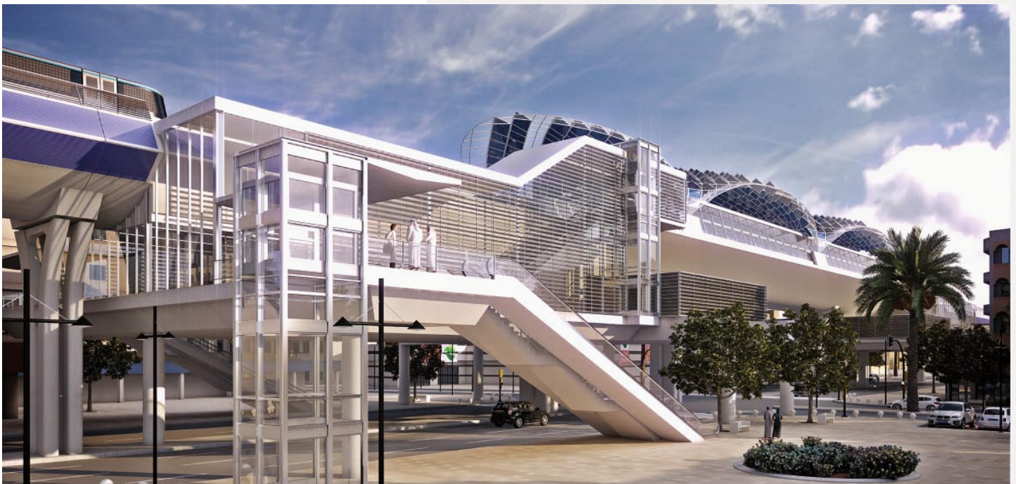
Riyadh Metro Project, Saudi Arabia
