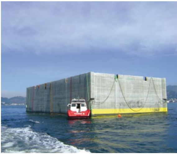
Towing of caissons in Brazil
