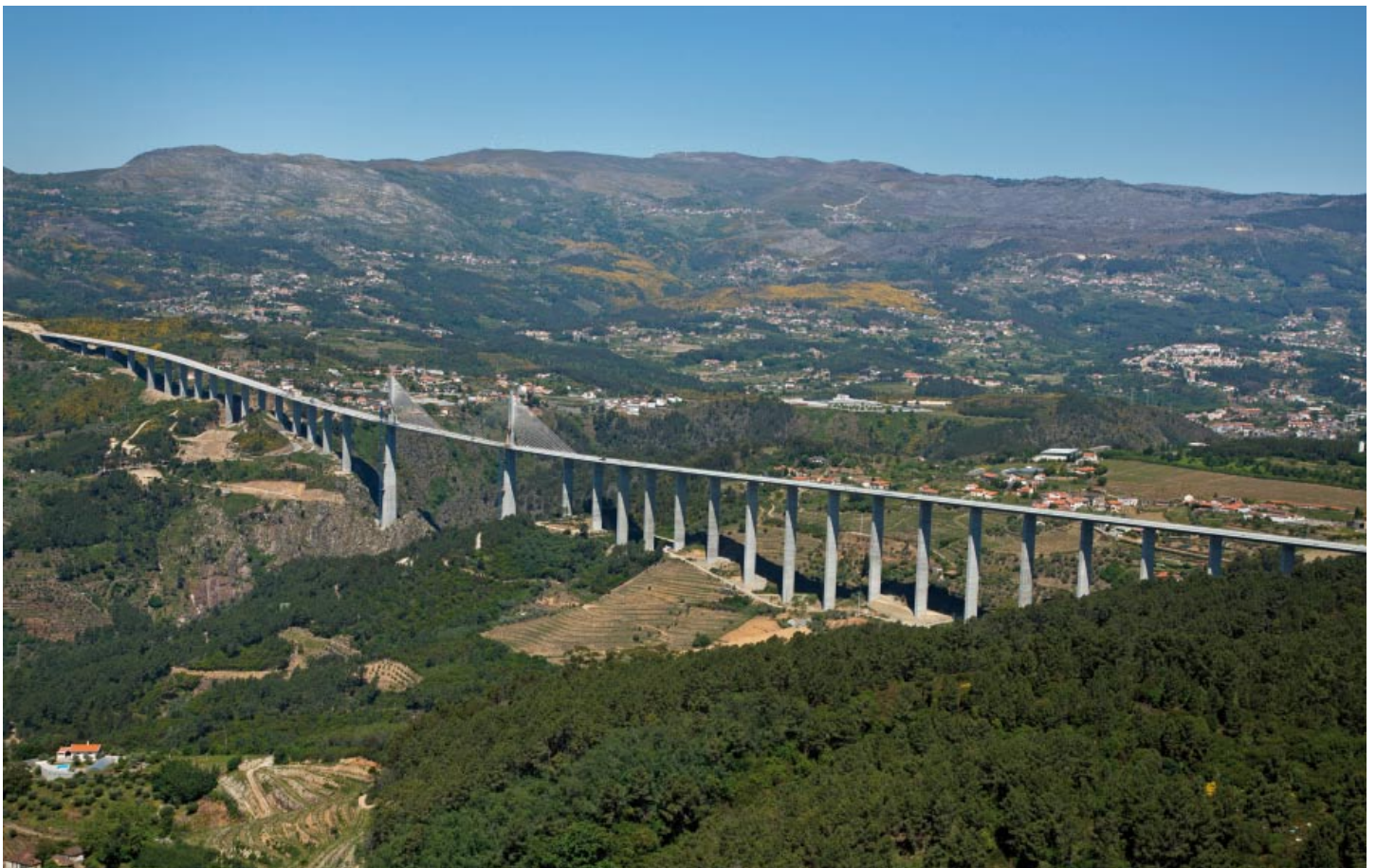
Do Cargo Viaduct at the Transmontana Motorway, Portugal
