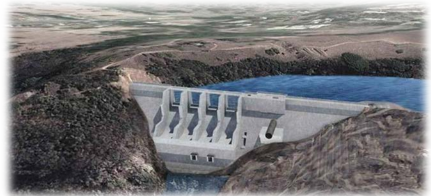
Chucas dam and hydro power plant (Costa Rica)
