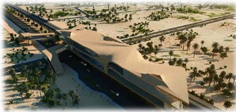
Doha metro (Qatar)
