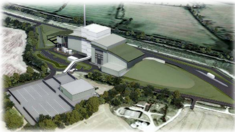
Buckinghamshire energy from waste start up in 2014
